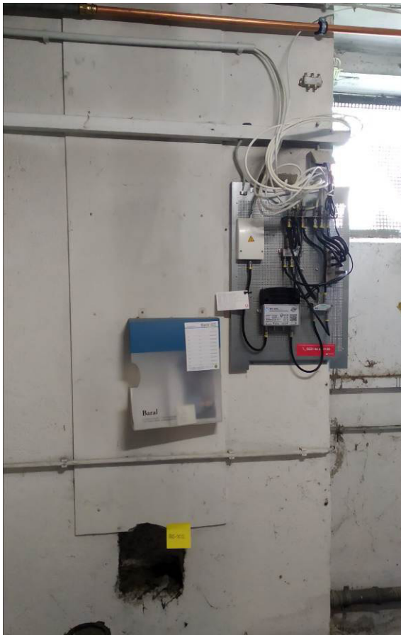
Asbestzementplatte Heizraum [BS102]
